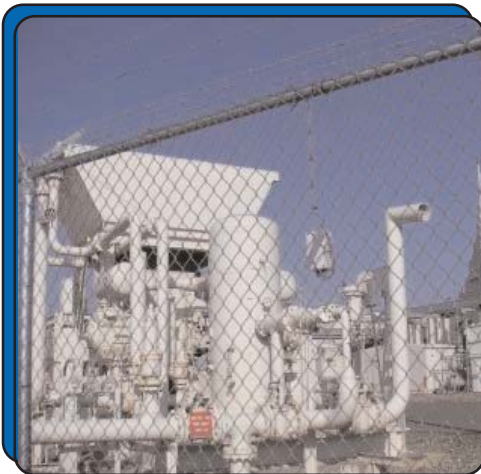
VIBRATION SENSOR VBS100 ELECTRICAL SUBSTATION
